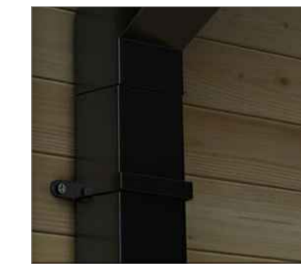
ALUMASC RAINWATER FLUSHJOINT ALUMINIUM RECTANGULAR RAINWATER PIPES WITH CONTEMPORARY RAINWATER HEADS REF.CP25.30.40HOP (OR SIMILAR), COLOUR: RAL 9017M BLACK.
